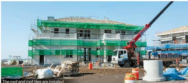
The roof and roof tiles are installed.
